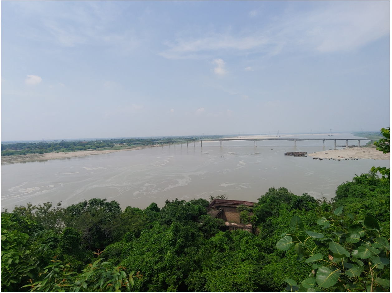
Figure 34 View of Ganga from Chunar Fort
