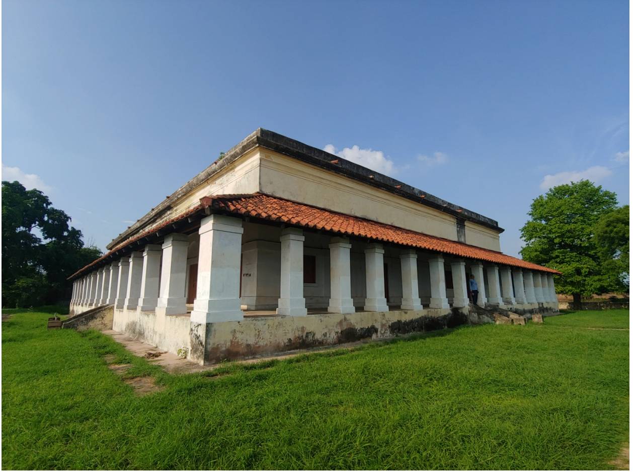
Figure 31 Warren Hastings' Bungalow at Chunar Fort
