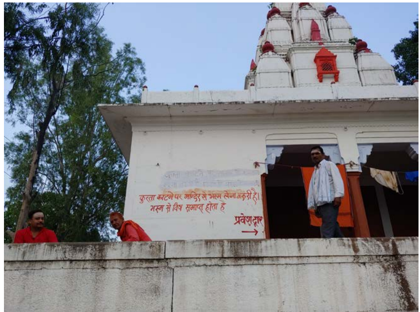
Figure 84 Mukteshwar Nath Temple, Vindhyanchal
